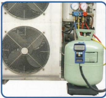
Charging for A/C System 空调系统加注
